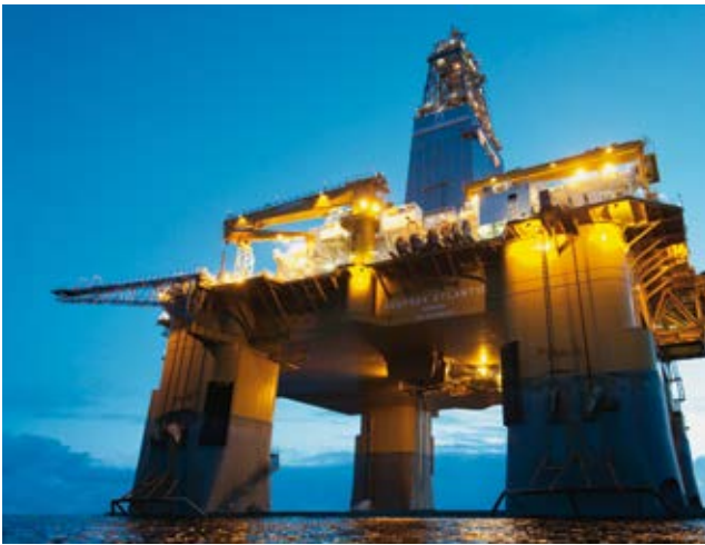
Safe power distribution on the drillship – with SIVACON S8
