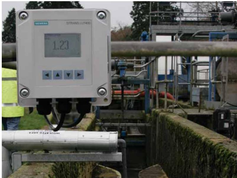
The SITRANS LUT400 can be installed in a variety of mounting locations, including on DIN rails, pipes, or walls.
