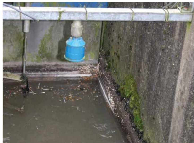
The new SITRANS LUT400 series controllers are compatible with all Echomax transducers, so operators had no need to replace their existing transducers.
