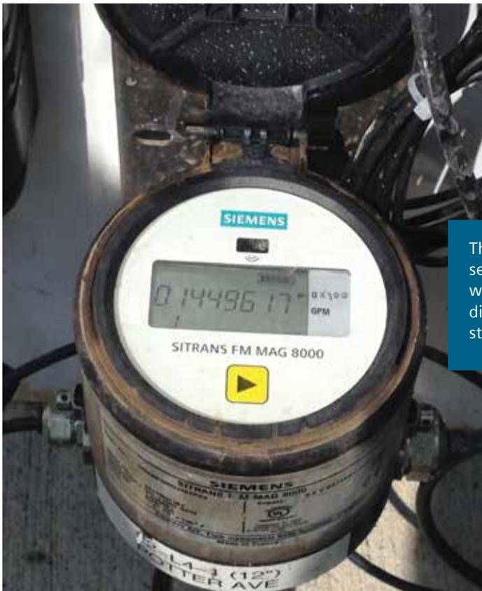
The transmitter can be remotely mounted, as seen in Figure 2. This, according to Kolkebeck, was an important feature, because of the difficulty of entering a manhole located in the street.
