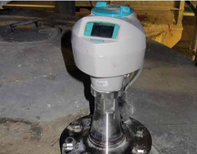
Installing the SITRANS LR250 was easy and Albemarle now has reliable, high-performance continuous level measurements on their process vessel.
