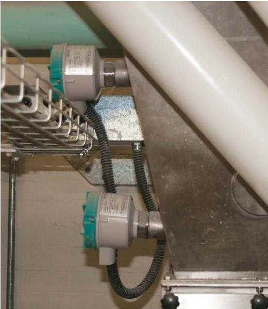
SITRANS LPS200 level paddle switches monitor high and low levels in the gluten hopper.
