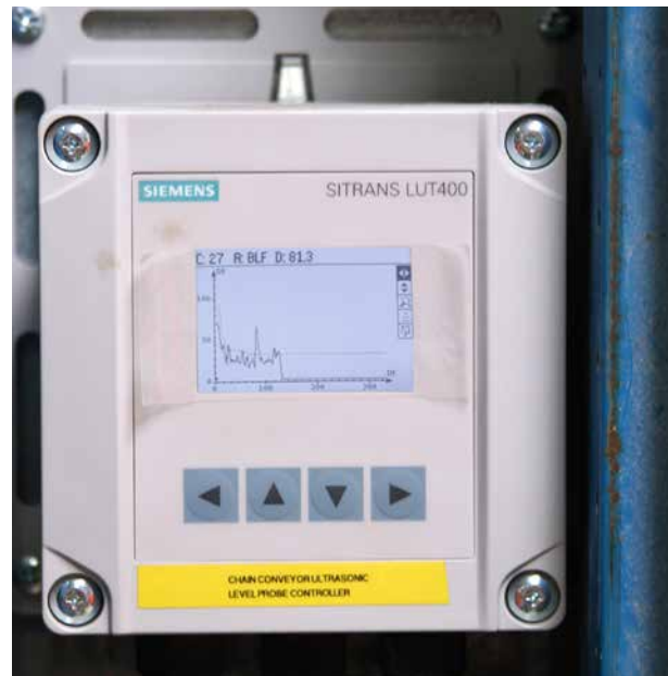
SITRANS LUT400 ultrasonic controller reliably monitors levels of clay moving from the intake belt conveyor to the shredder.
