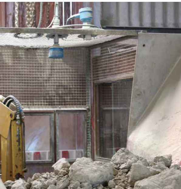
The Echomax transducer (left) relays continuous level readings to the controller, while the SITRANS ULS200 (right) provides a high-level alarm if clay reaches a certain point above the shredder.
