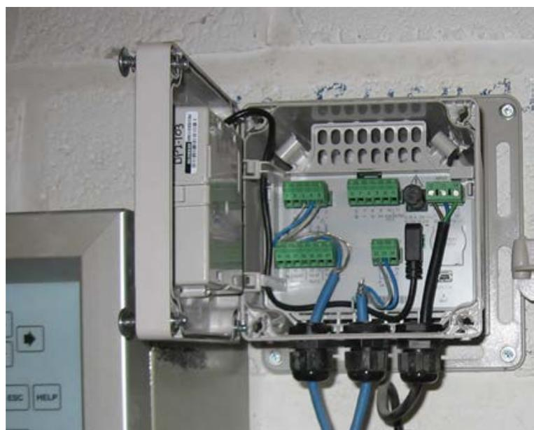
Installation and setup was simple with the controller's removable terminal blocks for ease of wiring and the convenient 1/4 turn fasteners.
