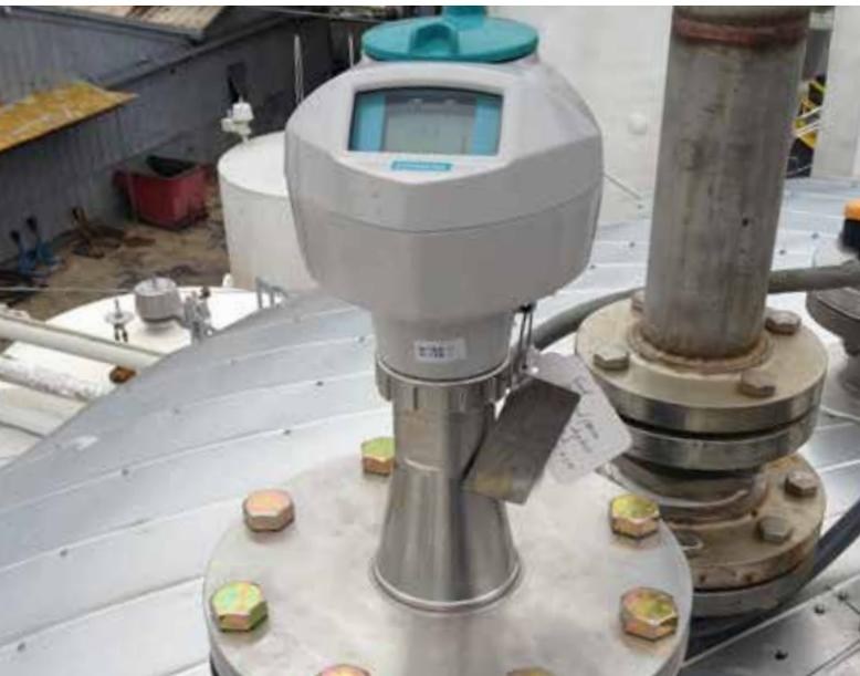
Installing the SITRANS LR250 was very easy on one of the chemical storage tank's existing process connections.
