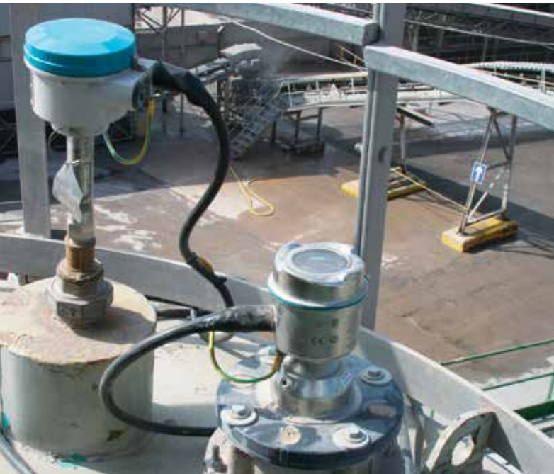
The 78 GHz SITRANS LR560 radar transmitter (right) provides continuous level readings of fibre, while SITRANS CLS300 (left) gives high-level alarming.
