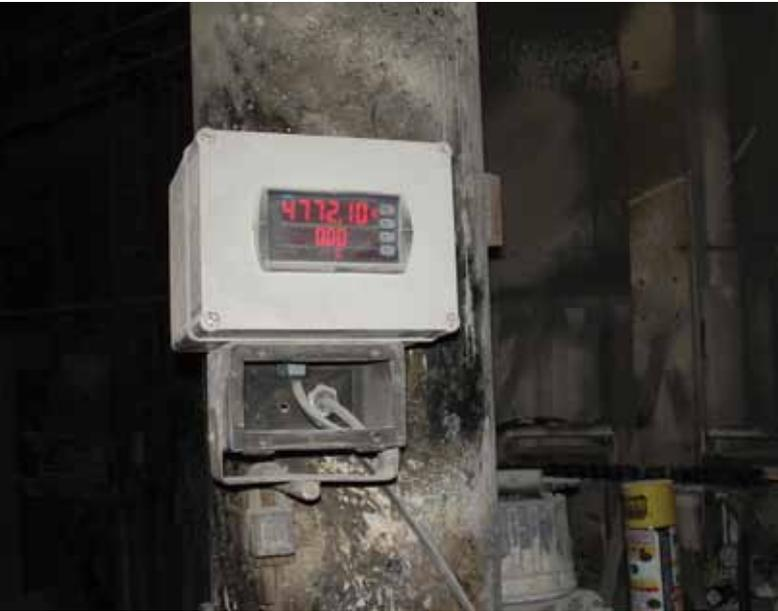
The SITRANS RD300 remote display monitors the flow rate and total amount of cooling water used in the harsh steel plant environment.
