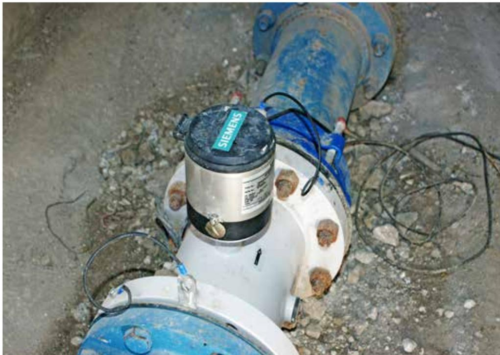
More than 100 SITRANS F M MAG 8000 electromagnetic flowmeters are now in operation across the various water distribution zones managed by Aguas de Saltillo.
