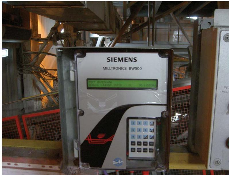
The belt scale relays information to the Milltronics BW500 integrator, which provides operators with belt speed, material flow rates, and other crucial information.
