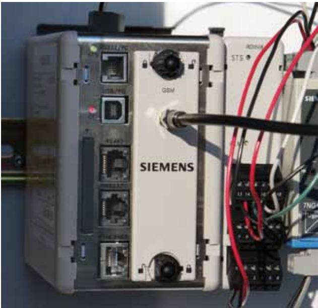
Level transmitters are connected to the SITRANS RD500 remote data manager.
