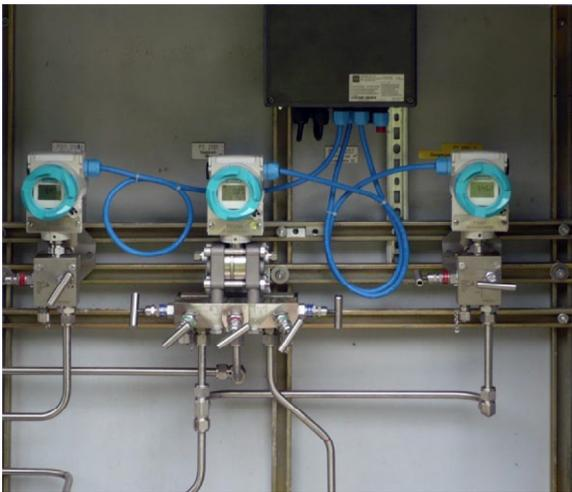
**The Gas Compressor Station Uses Pressure Transmitters with SIL2 Safety Loop Capability. SIL3 Is Possible In A 2oo3 Configuration, as Shown Here.**
