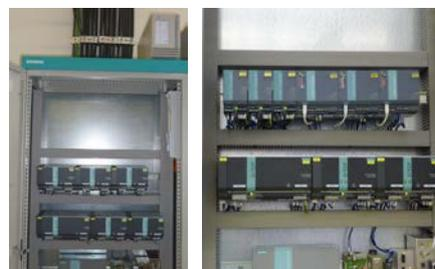
*Figure 1: With this control cabinet for controlling a crane system, an AC UPS which had to be mounted on top of the cabinet because of its size (photo left) was replaced by three DC UPS modules. Since the more compact SITOP PSU300M 24 V/ 20 A generation of power supplies was used at the same time, all three power supplies even fitted together with the three SITOP UPS500S 15A/5 kW modules on the same DIN rail.*
