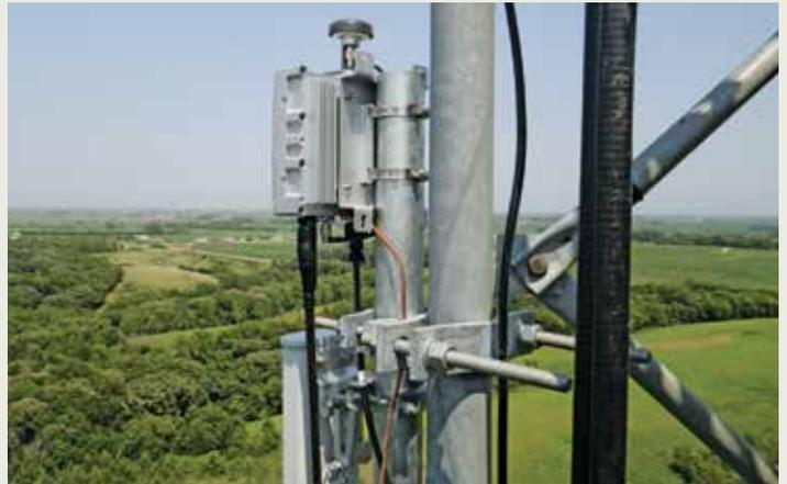
Connected to the RX1500 are Siemens RUGGEDCOM WIN 7237 outdoor wireless base stations that comply with the IEEE 802.16e WiMAX standard. The CCPPD obtained an FCC license to use the 3.65 GHz radio frequency, which is just one of nine spectrum options the WIN family offers.
