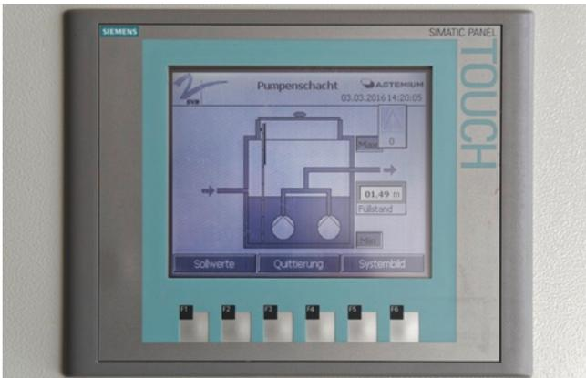
The touch panel allows cost-effective operation and monitoring of the pumping station on-site.
