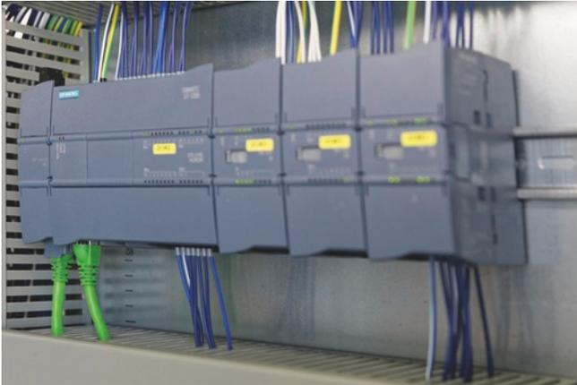
Compact automation solution with potential for retaining the system: With the aid of the communications processor CP 1243-8 IRC (far left), the SIMATIC S7-1200 controller can be connected seamlessly to the existing telecontrol system.
