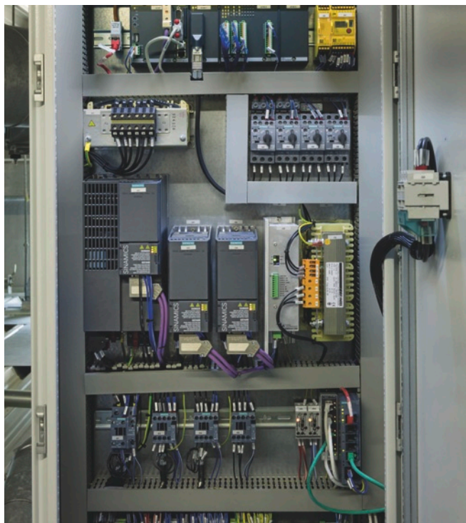
The control cabinets at Aesica were completely rebuilt.
