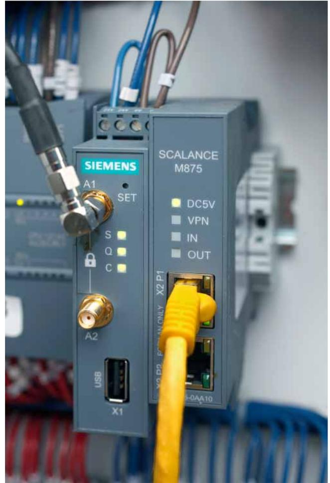
Waste Harmonics relies on a Siemens solution with the 3G cellular router SCALANCE M875 and the PLC SIMATIC 57-1200.
