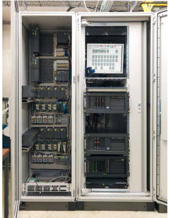
All threads of the redundant high-end automation solution come together in the control cabinet of the waterworks. The Siemens remote-control components are also installed here.
