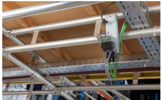
The link between the RFID readers and the central controller is provided by PROFINET communications modules SIMATIC RF180C – here with the particularly easy to install push-pull terminal block with two RJ-45 jacks.
