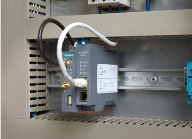
Fast and secure (thanks to the firewall and VPN with IPSec) WAN communication is an essential feature of the new SCALANCE M875 UMTS router from Siemens.
