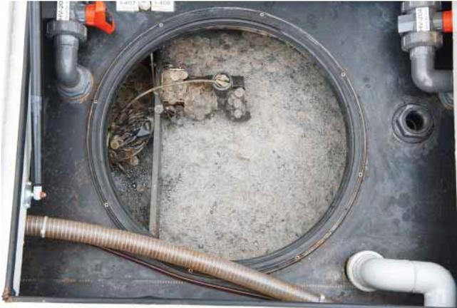
The „moving bed“ of the bioreactor is formed by so-called chips, which float freely in the containers and are used for the bacteria biology.
