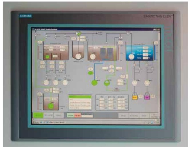
Thanks to the fast wireless transmission via secure UMTS router, the treatment plants can be operated and maintained both locally and remotely.
