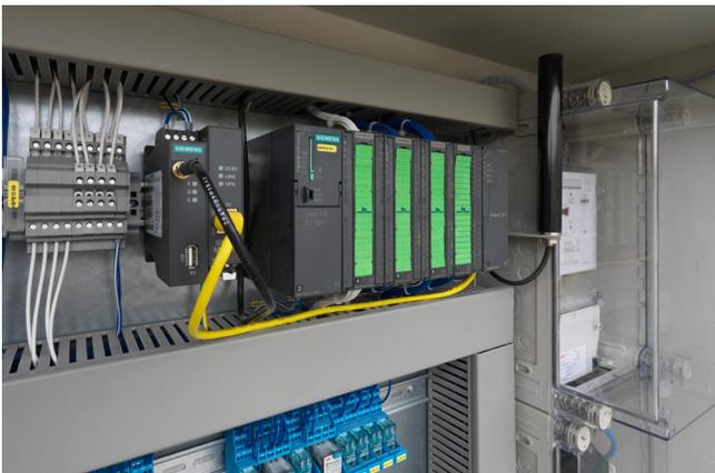
The remote stations are always connected with the control center via GPRS to transfer process data, such as the water level.
