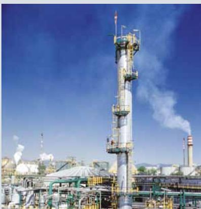
*Zimpro® wet air oxidation system uses oxygen to treat high strength styrene monomer and polyol wastewater at Repsol YPF, Tarragona, Spain.*
