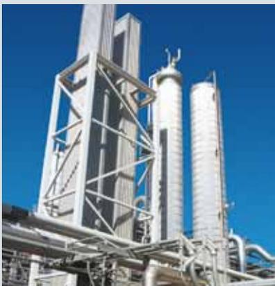
*Zimpro® wet air oxidation system treats the spent caustic effluent generated by the world's largest naphtha steam cracker at the BASF ethylene facility, Port Arthur, Texas.*
